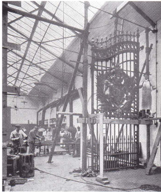
One of the centre gates under construction in the workshop of the Bromsgrove Guild, c.1905–6.
