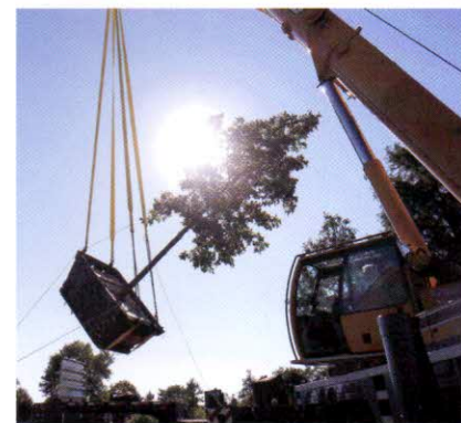
Each memorial swamp white oak tree lived in its own box for four to five years before being installed by crane on the plaza.
